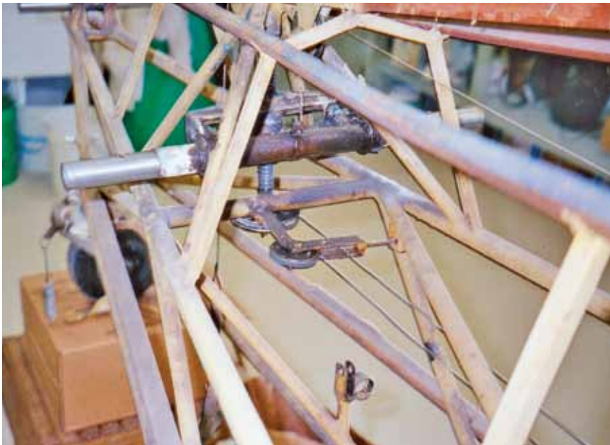
Close-up view of the old trim system.
